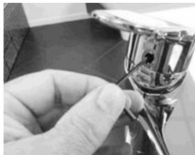
Use Allen Key to tighten or undo
